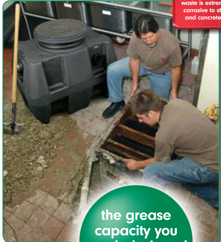
Photo Series: replacement of failed steel interceptor (Chuck E. Cheese)
