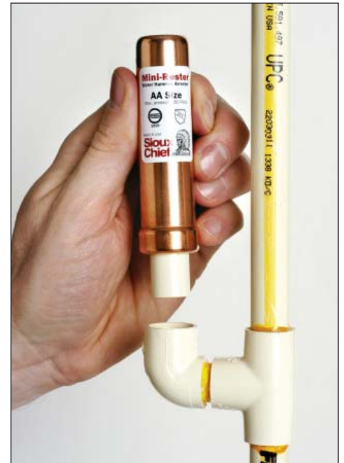
Male CPVC arrester fits directly into female fitting, eliminating extra joints.
